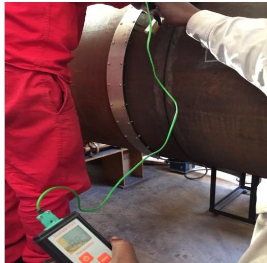
Inter pass temperature monitoring
