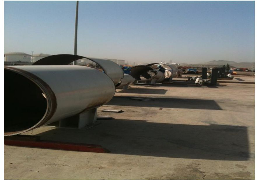
Laying the pipe for welding
